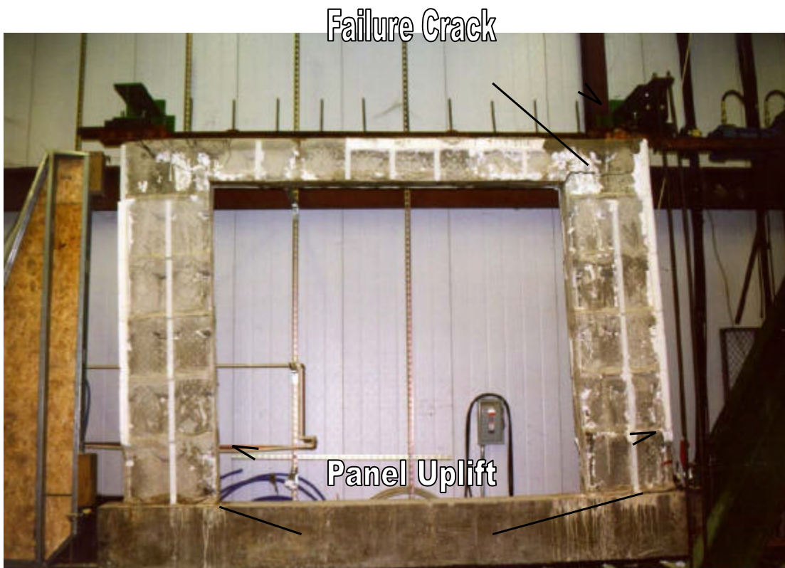
Figure 10 Final Lateral Displacement of Waffle No. 3 Wall Specimen
