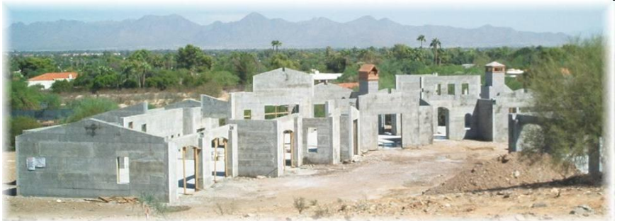
Home Under Construction
