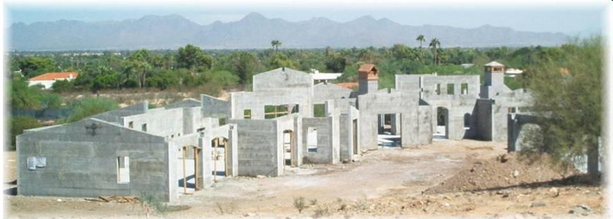
Home Under Construction
